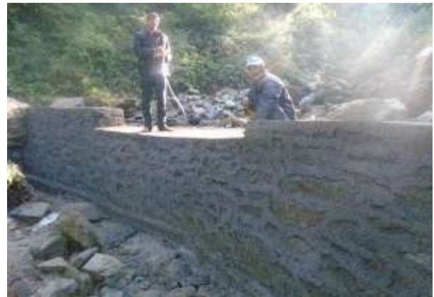
Measuring the actual quantity in field at Panchakanya
