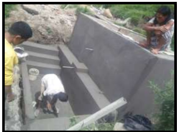
Drinking water tap construction
